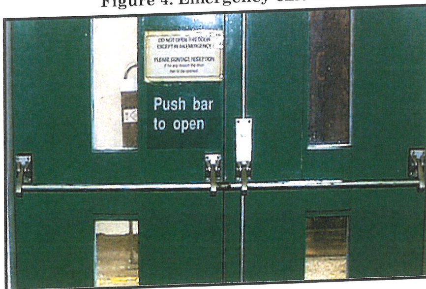
Figure 4: Emergency exit doors
